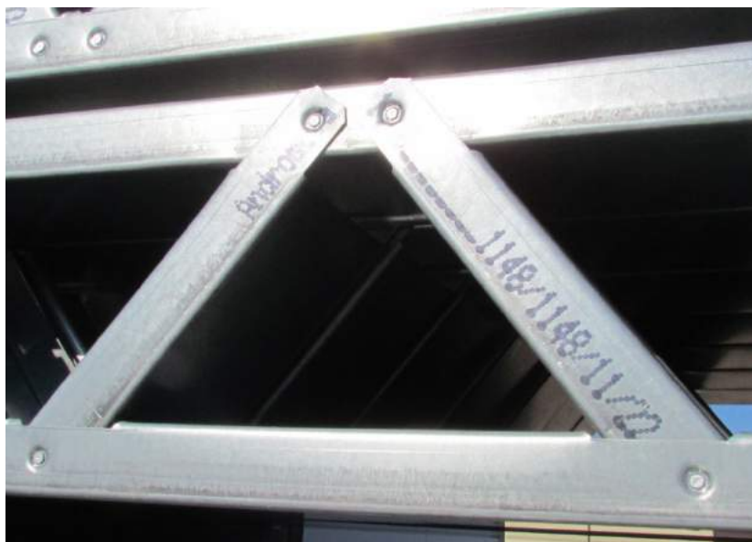
0050 Swaged corner with 2 lifting holes
